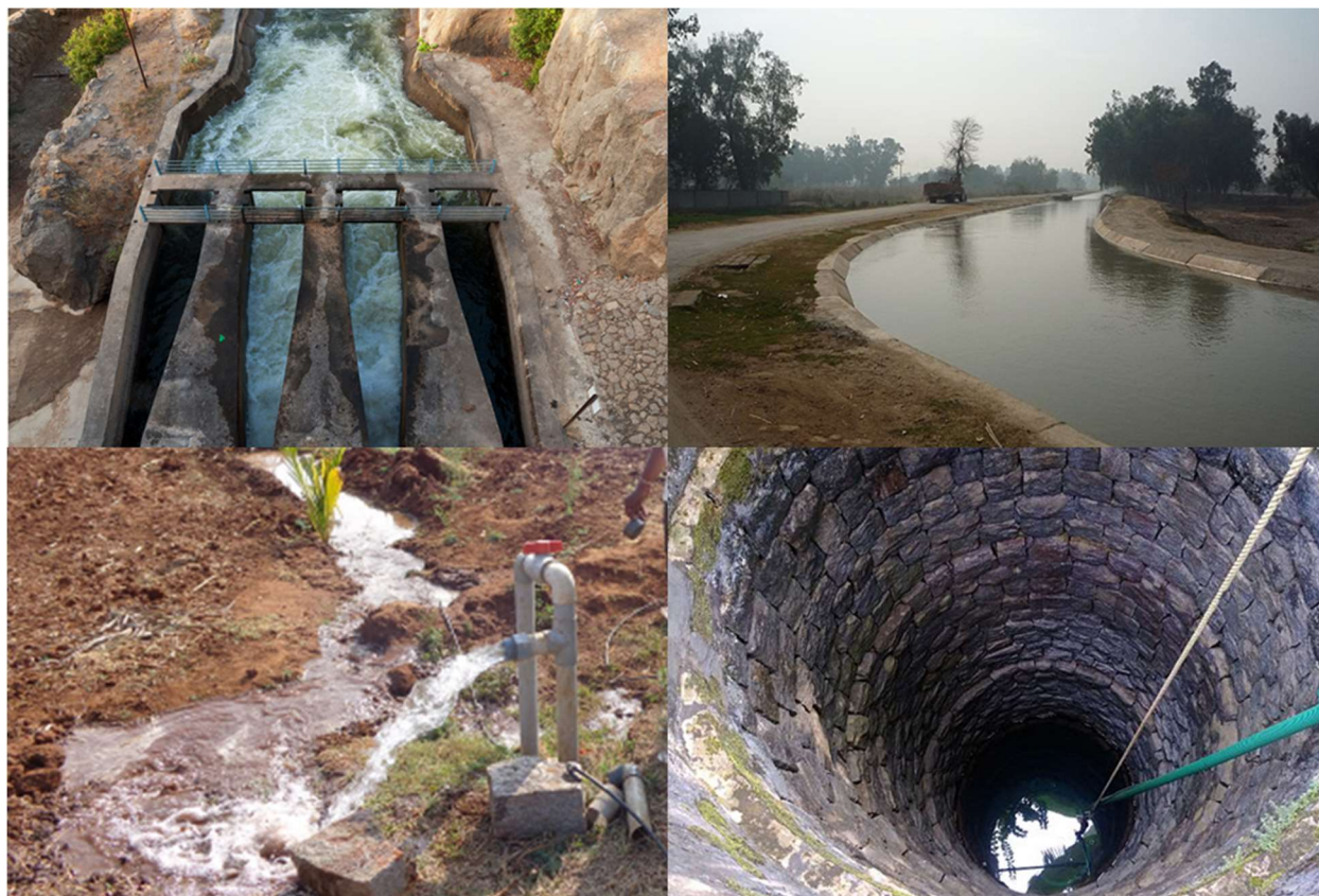
Water storage structures used in irrigation in non-monsoon months. (Clockwise from top) Check dam, canal, borewell, dugwell
